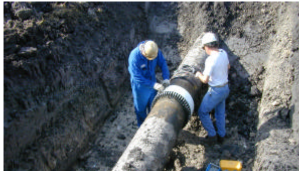
Figure 6. Pipeline inspection of “bell holes” and unpiggable pipe sections (Teletest®)
